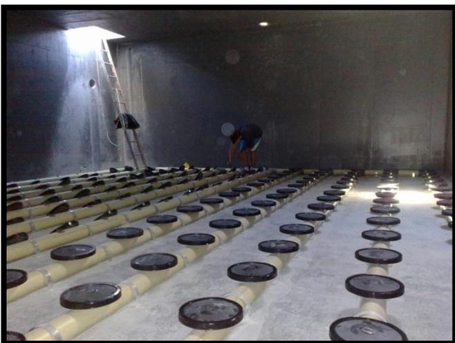
When comparing different aeration techniques, oxygen transfer efficiency is an important yardstick. Aeration systems are usually rated by the mass of oxygen transferred per kilowatt hour. The more oxygen transferred per kilowatt hour, the more energy efficient the system. Because it is difficult to get dissolved oxygen into the bioreactor a lot of energy is lost in the process of oxygen transfer. Big bubbles do not necessarily translate to dissolved oxygen.
